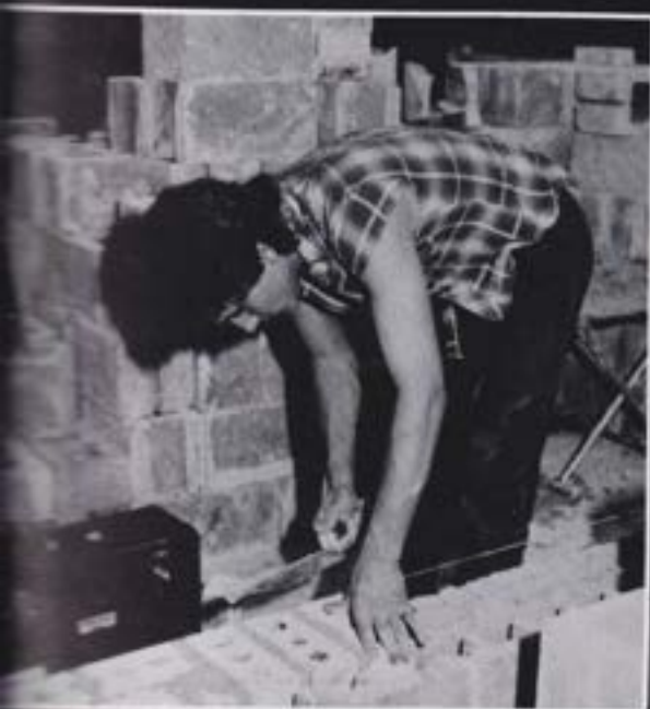
(TOP RIGHT) Mr. Jerry Cook, Instructor, observing a student building a brick lead. (ABOVE) Officers: L to R — B. Sturgill, Pres; M. Bloomfield, Treas; J. Bentley, Sec; K. Smith, Sgt. Arms.
