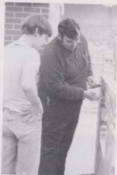
(ABOVE) Mr. Greg Compton, Instructor, showing Jeff Mundhenk how to strike mortar joints.
